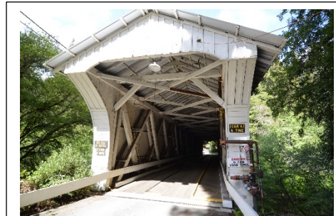
The Powder Works Bridge, built in 1872, spans the San Lorenzo River in the San Lorenzo Valley. The bridge became a National Landmark in 2015 due largely to its use of a Smith truss, a nationally noteworthy timber truss type developed by Robert W. Smith.
