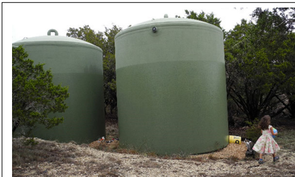
The Fire Code requires a 10,000-gallon fire water storage tank for a new 4,000 square foot home that relies on private water. Although dimensions vary, a typical 10,000-gallon tank would be 12 feet in diameter and 13 feet tall. The 10,000-gallon requirement for a home may also be met by two 5,000 gallon tanks.
